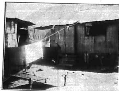
Dilapidated and insanitary Asiatic housing. Demolished under Magistrate's order, 1924.
