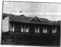
Improved type of Asiatic dwelling. The result of a demolition order and reconstruction.
