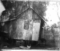
Insanitary and dilapidated Asiatic housing.
