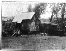
Insanitary and dilapidated Asiatic housing.
