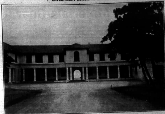
Main entrance to the reconstructed Government House, Mombasa.
