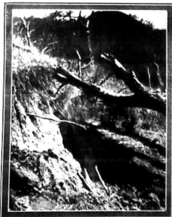
A clear indication of subsidence.
