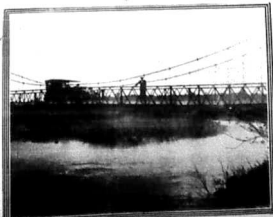
Photo: (1) by G. W. Harvey, Nairobi. The Yala River Bridge.
