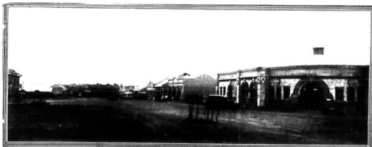
A section of Kibaha's Main Street.
