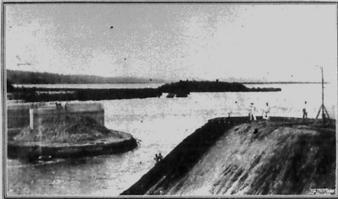
The new link between Malindi Island and the Mainland. The gap to be bridged between the approaches.
