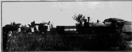
The locust train which is being used on the Main Line and on the Voi-Taveta Branch. The pump tank and the manual pump at work can be seen.
