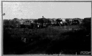
A few of the lorries being held up by the collapse of the Tsavo Bridge. This is indicative of the road traffic of this route.
