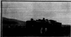
The engine which left the rails at Longnot Station on April 26th being jacked up prior to replacement on the line. A wire line was built in remarkably quick time in a direction to permit the passing of other traffic.
