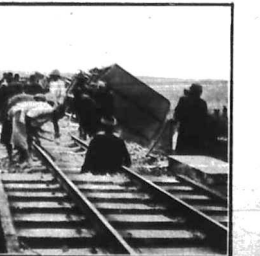
REPAIRING THE DAMAGE.
