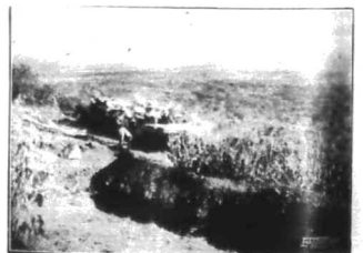
A TRENCH ON LONGIDO HILL. Photo by M. R. S. from Longido, B.E.A.
