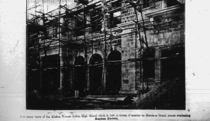
Recent views of the All India Vijnan Indian High School which is now in course of erection on Mombasa Island, almost overlooking Mombasa Harbour.
