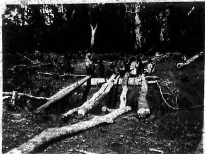
Bridge Building - Laikipia
