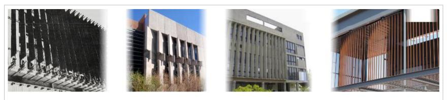
Figure 2-6:illustrations of vertical shading devices in use, Source: Arch daily 2020: Facades and solar control, Brise Soleil Systems for residential, commercial, corporate, hospitality
