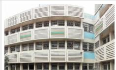
Figure 5-5:horizontal vented concrete shading on N block: Source: author
