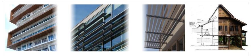
Figure 2-5:illustrations of horizontal shading devices in use, Source: Archdaily2020: Facades and solar control, Brise Soleil Systems for residential, commercial, corporate, hospitality
