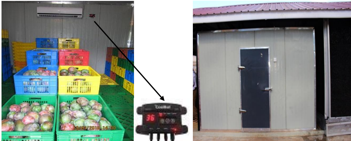
Figure 3.2: The Coolbot™ cold room with crates of mango fruits (Source: Karurumo Smallholder aggregation and processing center, Embu County)
