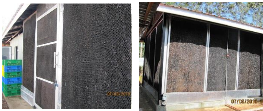
Figure 3.1: Front and rear view of Evaporative Charcoal Cooler (Source: Karurumo Smallholder aggregation and processing center, Embu County)
