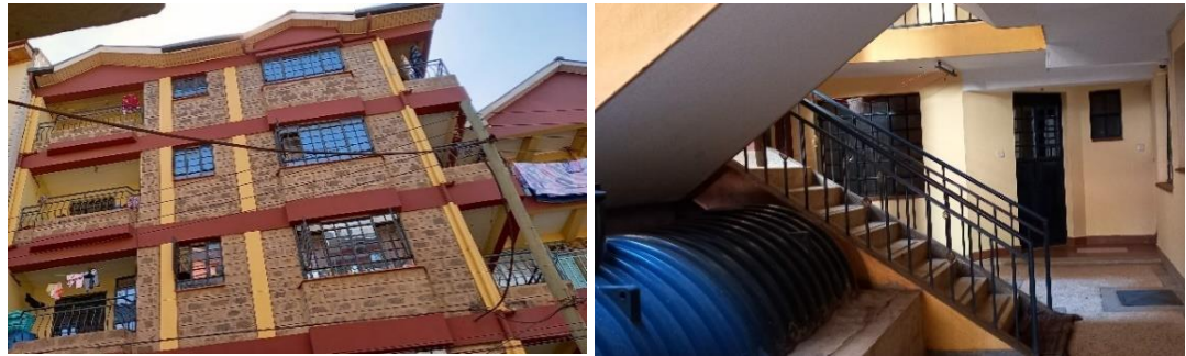
Figure 48 Building 2 front and atrium view showing the balcony type, the railing. Source; Author, 2021.
