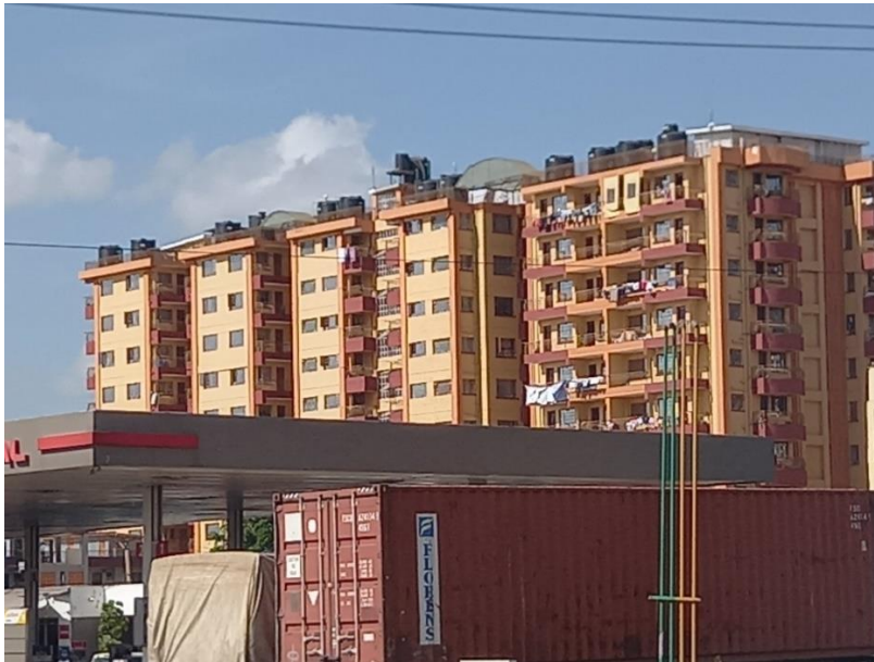
Figure 2 High densities driven by market forces, high land prices and demand for low-cost houses have reduced energy efficiencies in many neighbourhoods. Source; Author 2021, Thika, Kenya
