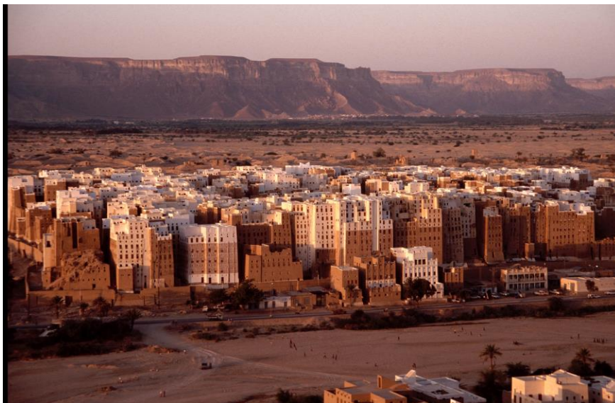
Figure 6 Yemeni 16th century apartments made from mud brick. Source; (Goran, 2021).
