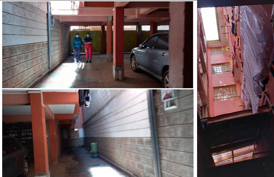
Figure 51 Photos of building 3 showing atrium and ground floor spaces. Source; Author 2021.
