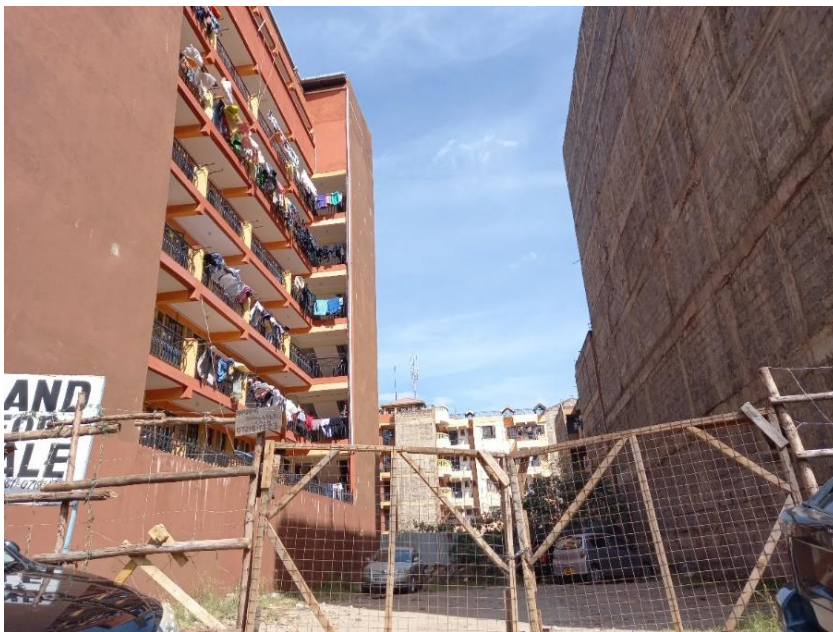
Figure 29 Roysambu buildings are built without consideration of future upcoming developments. Source; Author 2021
