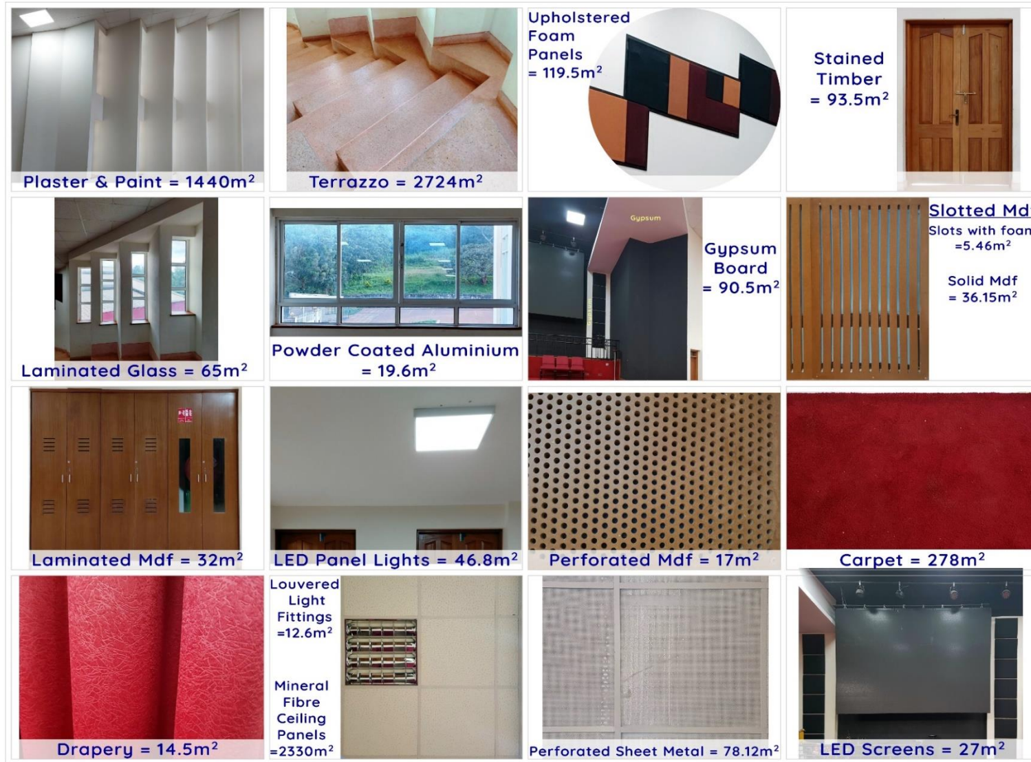
Figure 55. CITAM Ngong: Surface finishes
