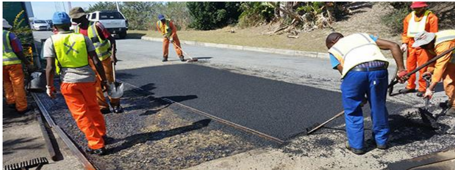
Plate 2-3: Section of the Northern Corridor under Maintenance
