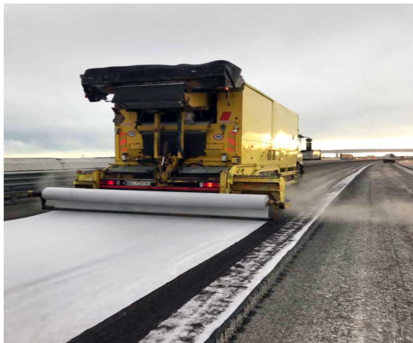
Figure 2-5: Laying of SAMI (Marcuzzi, 2022)
