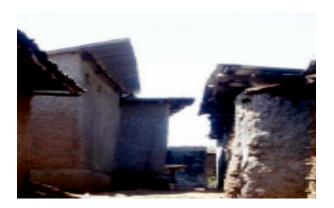
FIGURE 5 The mud-plastered wooden skeletal structures of Kibera slums Source: JKUAT Cohort 2015
