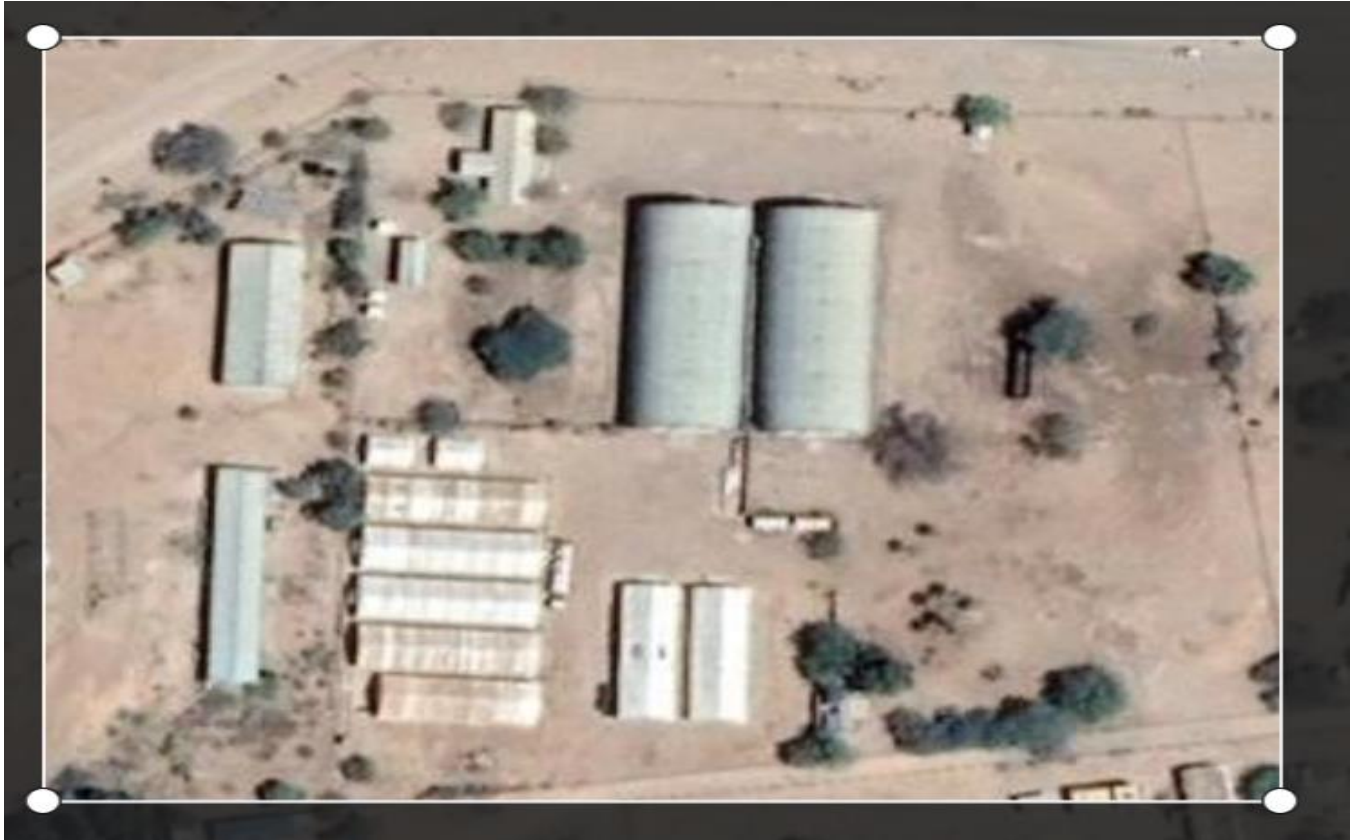
Image 1 35 Picture of the Cereals storage facility.
