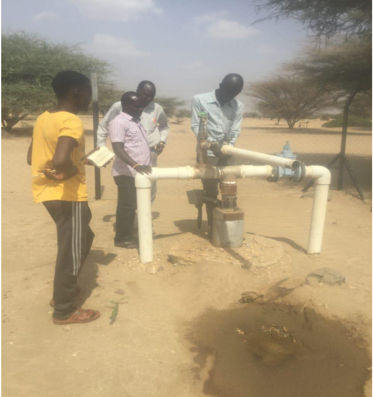
Image 1 41 Picture of a borehole in Turkana Central
