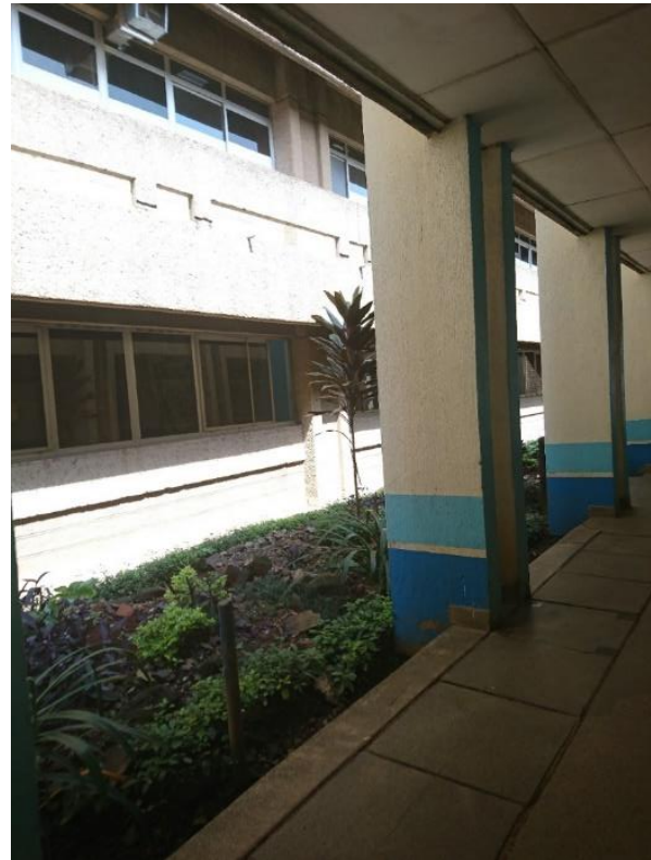
Figure 3-1: Kenyatta National Hospital Walkway adjacent to Maternity Wing (Source Author)
