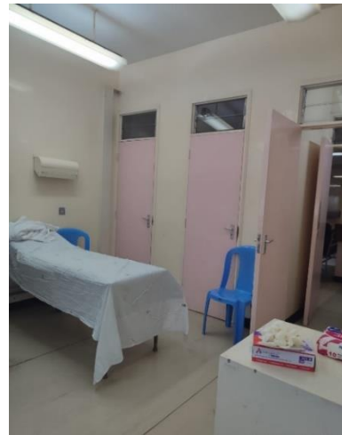
Figure 5-4: KNH, antenatal clinic: note the high-level louvre windows and larger window panels at sill height of 1000mm
