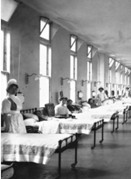
Figure 2-2: Victorian hospital window with a tall sash and a top hopper window operated by a crank e control at nurse height. (Fordham & Thomas, 1996).
