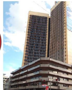
GPO Telposta towers
