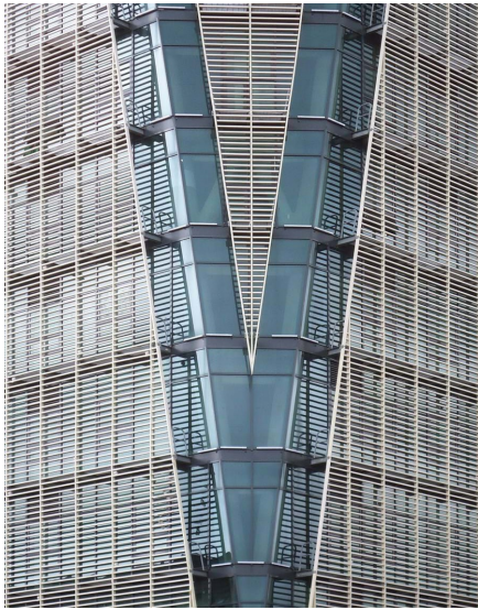
Fig2.57. Sun shading solution to the glass facade of Britam Tower, Nairobi.
