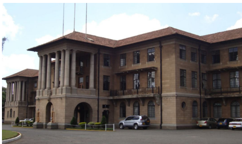
Fig4.27 Railways headquarters front facade
