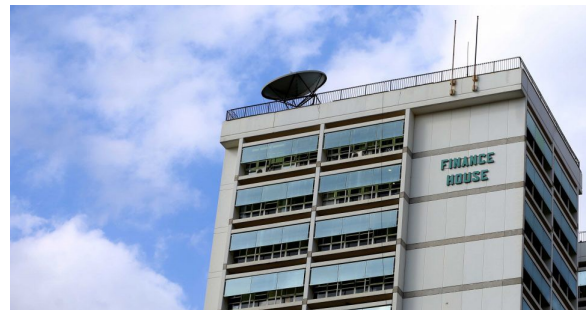
Fig2.9. Horizontal sun shading devices at Finance House, Nairobi. Type J according to fig. 2.7 Source: Flickr.com
