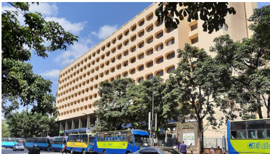
Fig5.4. Recessed windows of Kencom building facade act as secondary sun shading feature.
