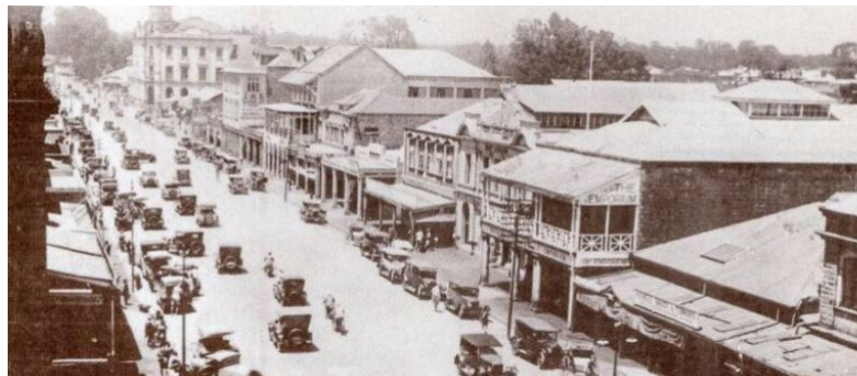
Fig 4.24. Nairobi's Government road in 1927 showing Khoja mosque, the tin buildings of the previous era and newer storied masonry buildings.
