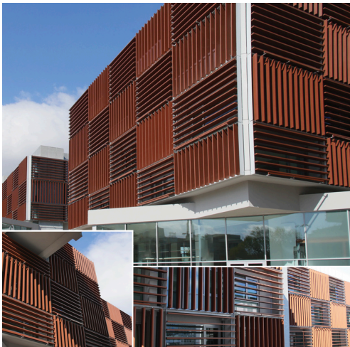
Fig5.5. Variations of timber brise soleil on a building showing use of different materials and kinetic sun shading devices in use in the Western world.
