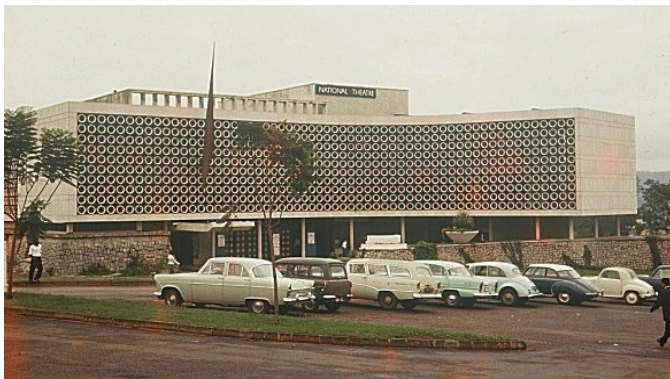
Fig2.13. Circular egg crate shading on Uganda National Theatre and Cultural Centre in Kampala Uganda designed by Peatfield & Bodgener in 1956. Source: https://3rdworldarchitecture.wordpress.com
