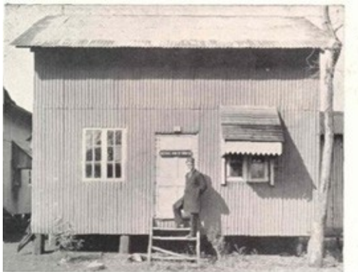
Fig 4.17. Bank of India in 1904 on Government Road. Source: Buildesign.co.ke
