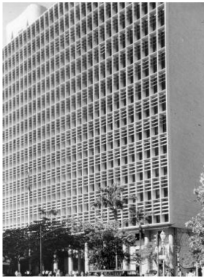
Fig 2.35. Sun shading devices on the Ministry of Public Health Building in Rio.
