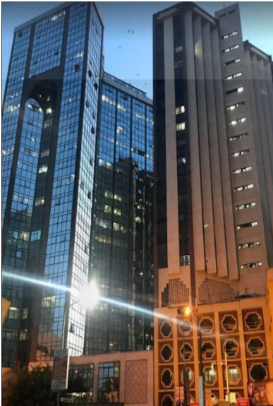
Fig 4.37. Image of New glass buildings in Nairobi..
