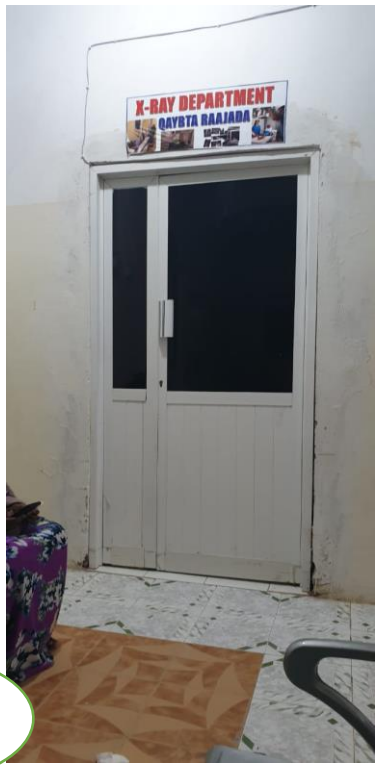
Image 4: Entry door to x-ray room which is made of aluminium
