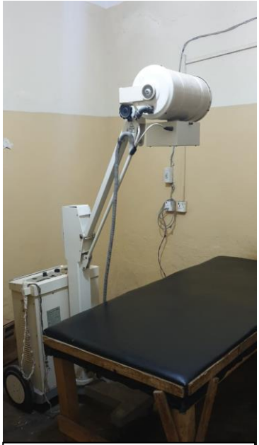
Image 2: Xray room without control panel
