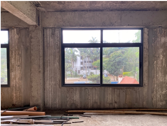
Figure 4.2.2:5 Precast wall panels used on an active site.
