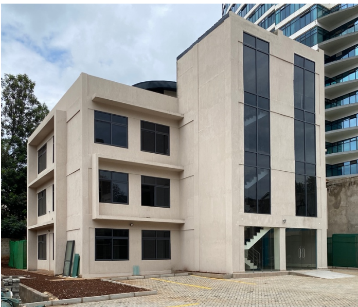
Figure 4.2.2:6 A building with precast wall panels used for all walling works.
