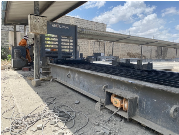
Figure 4.3.2:1 Precast beams OSM facility.
