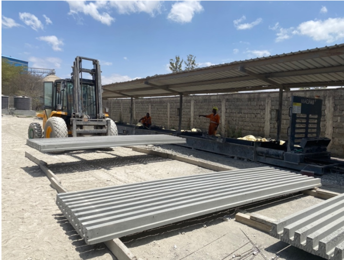
Figure 4.3.2:2 Precast beams transported to cure within the OSM facility.
