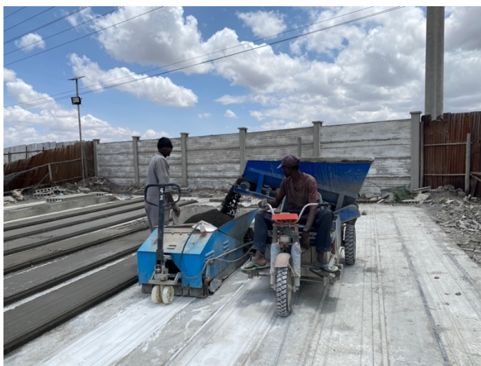
Figure 4.2.8:1 An offsite fabrication facility for wall panels.
