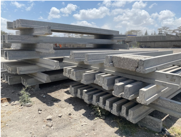
Figure 4.2.2:4 Precast beams and block at an OSM site.
