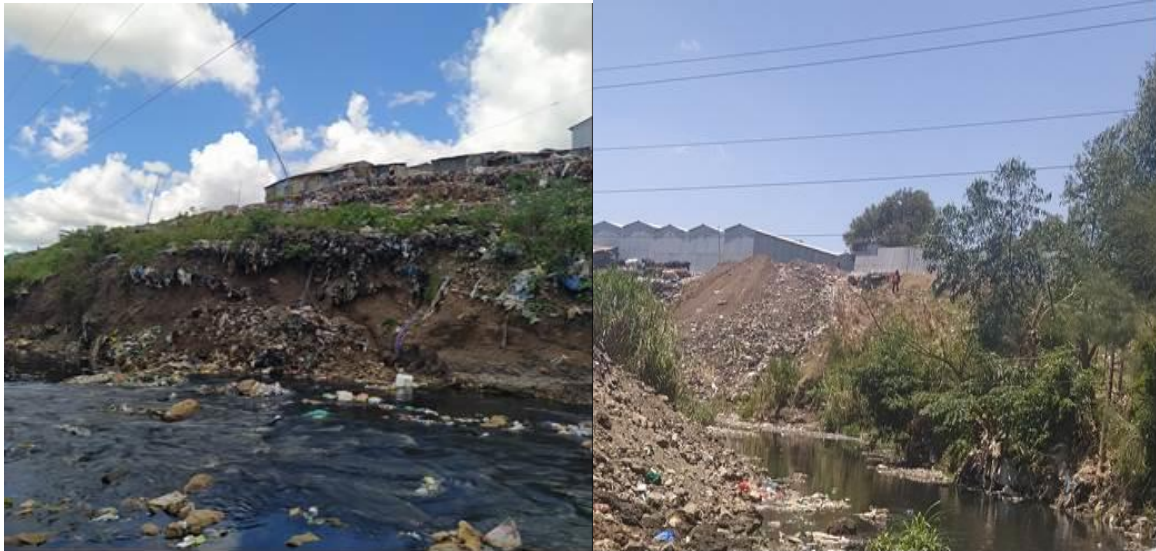
Plate 20: Informal settlements and soil dumping at Outering bridge Source: Field data (2021)
