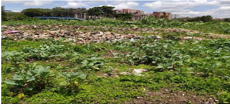
Plate 7 : Solid waste dumped in the encroached part of the dam Source: Field data (2021)
