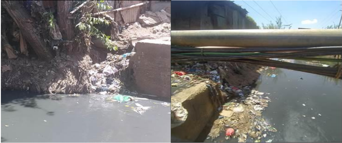
Plate 9: Open drain discharging domestic effluents into Ngong River at Mukuru Kayaba, dry season (Blackish river water) Source: Field data (2021)
