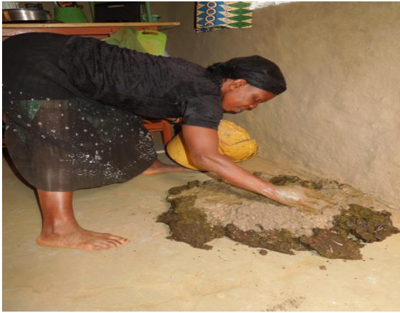
Plate 2-3: Step 3 -Mixing the materials slowly with water (Google)
