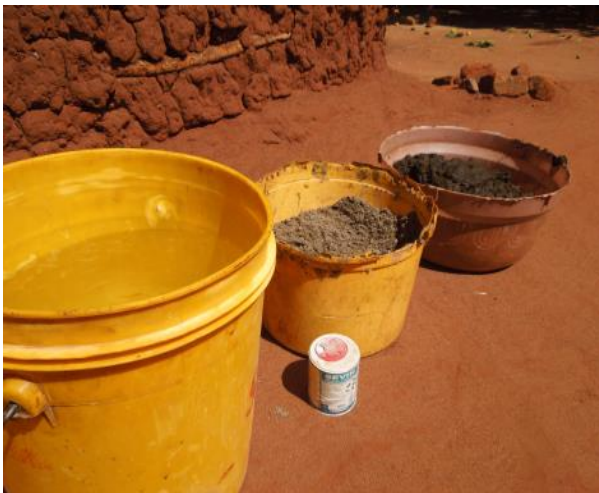
Plate 2-1: Step 1 -Materials (Sand, FCD, Water & Dudu Dust) (Google)
