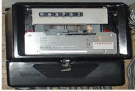
Figure 2.1: Electromechanical meter [3]
