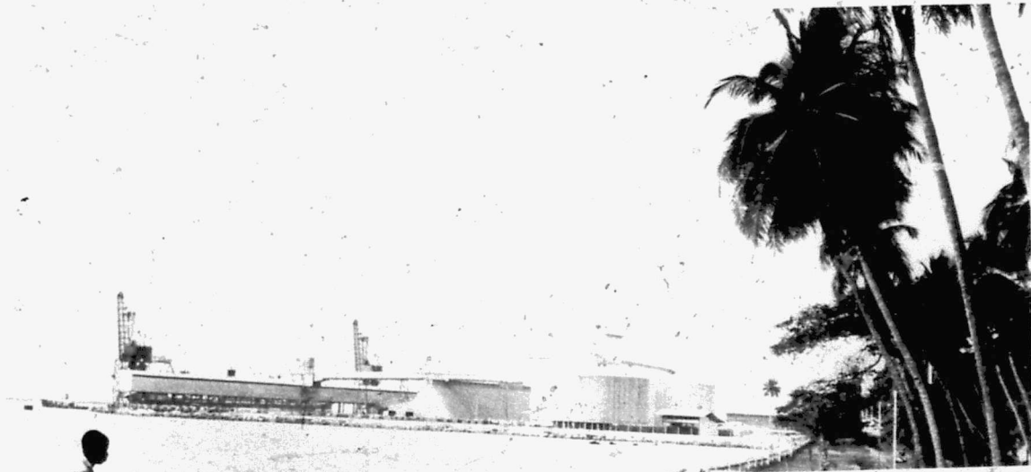
Conakry: A bauxite loading plant
