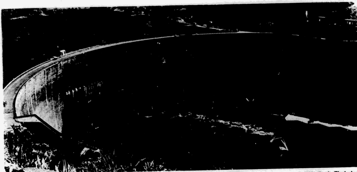
Kariba Dam, Zimbabwe: "SADCC is now interconnecting national electrical grids so that we can send power out of Kariba in Zimbabwe, for example, to deficit areas in Tanzania"
