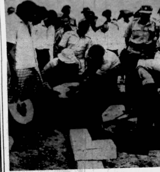
The North-Eastern Provincial Commissioner, Mr. Mburu, is seen laying the first stones of a health centre, which was being built by the Kenya Army to help bantu. Seen in the picture are several Kenya Army personnel.
