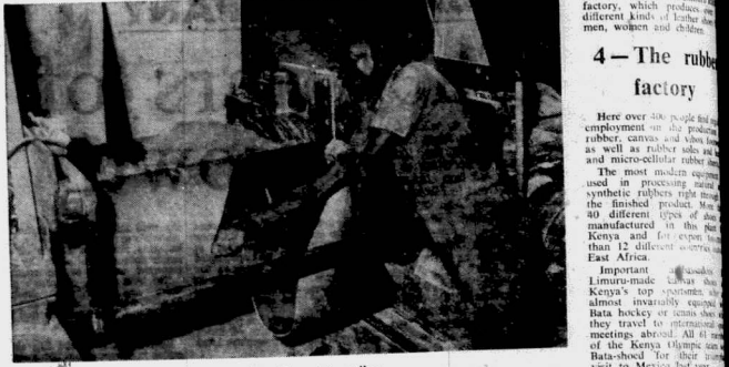
Operating the rubber mixing rollers.
