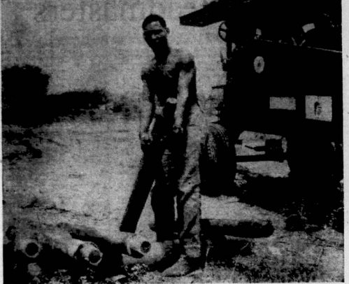
Sgt. A. K. Kabiah of the Kenya Engineers shows one of the massive drilling bits with which the unit has probed down more than 500 feet in search of water.
