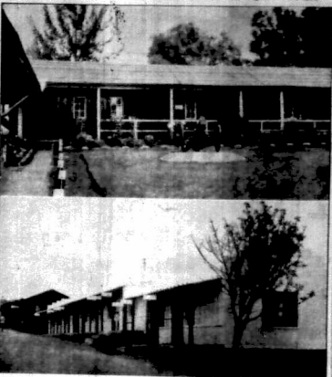
The Headquarters of East African Command situated near the new shopping centre at Hurlingham Road. The latest prefabricated buildings (above) centre with the older type (top). The 12 houses were presented to C.I.G. in 1955 by the 1st E.A.H.A.A. on disbandment.
