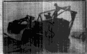
Road maker driven by a 15 ton tractor in the Western desert. (Official War Office Photograph)
