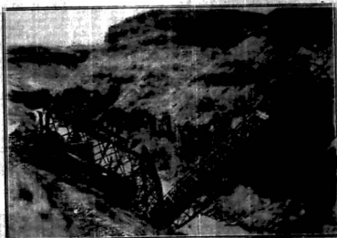
The Railway bridge over the River Awa sh after its destruction by the retreating Italians. (Official War Office Photograph)
