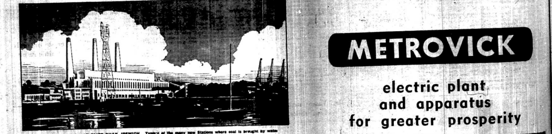
THE POWER STATION AT CLIFF QUAY, IPSWICH. Types of the many new Stations where coal is brought by water
