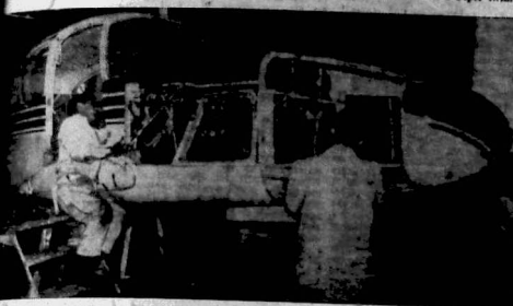
Engine shop at Wilken Aviation Ltd. handles all repairs and maintenance on Lycoming engines. One of the engineers makes a final adjustment after giving a thorough check to an engine.
