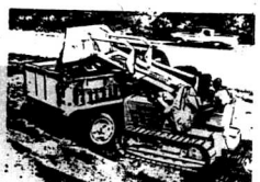
81 Loader on 440 Crawler
