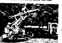
Work Lift and Log Loader on 440 Crawler
