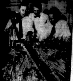
Mr. Basil Eastel, of the East African Railways and Harbours and Mr. (above), taking a shot for the film "Permanent Way" with one of the old rope railways built on the Kikuyu Escarpment at the end of the 19th century. Below, the real thing — the rope railway seen from halfway up the rope railway.
