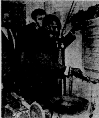
President Kenyatta seen paying the foundation stone of International Life House, Nairobi, yesterday watched by officials connected with the project. (Story in Page 5).
