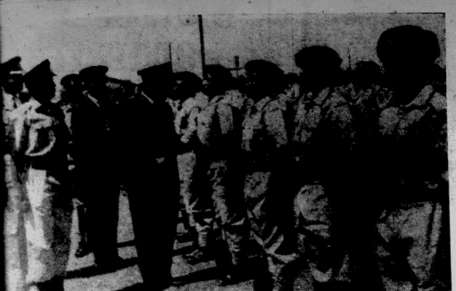
Hinga inspecting the passing-out parade of 592 boys and girls who had been under training at the Joint Youth Service Field Training Centre, Gilgil. He is accompanied by the Commandant of the Centre, Mr. S. R. Ujomo, and the Training Officer, Mr. Mutuse Kioko.
