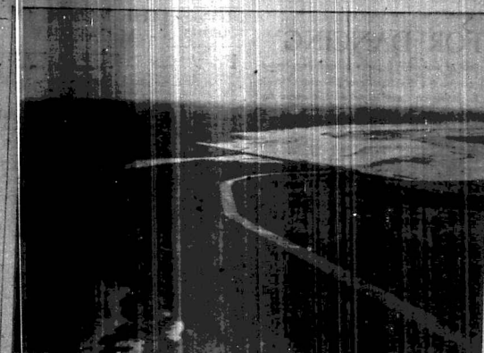
The Sudan Dam on the Nile Nile shows up the flood which for long in Sudan's long dry season. On the right is the main irrigation canal carrying over 10,000,000 cubic metres of water to the irrigated area of the Gezira plain.
