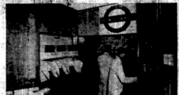
"Pneumatically" the control station of the large pneumatic tube system.
