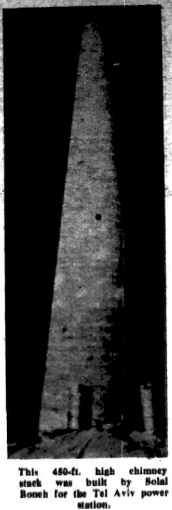
This 480-ft. high chimney stack was built by Solel Boneh for the Tel Aviv power station.
