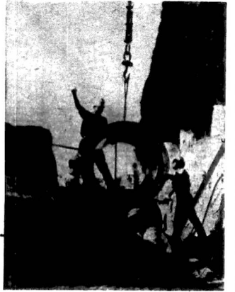
Laying a 36-inch pressure pipe made in Israel from asbestos cement, manufactured by Isabeh Ltd. of Nahariya. Asbestos products are exported to Kenya for projects such as low-cost housing and irrigation schemes.
