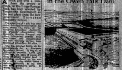
The question of a site has been... The Owen Falls Dam... The Owen Falls Dam... The Owen Falls Dam...
