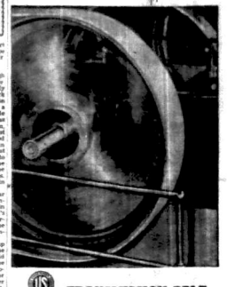
Transmission part brought from the Lane-Devon Engineering Co., Adams.
