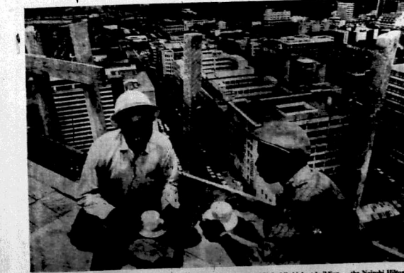
A tin break for two but not high one, although it is taking place on top of Nairobi's highest building — the Nairobi Hilton. These two workmen get a magnificent bird's eye view of the city as they relax over a cup of tea, while construction work more completion on the top floor.
