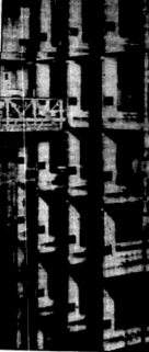
View of a robot car-park building of the type to be built between Queenway and Sergeant Ellis Avenue, Nairobi. It shows the parking floors and the spaces which are "filled" by the automatic lift in the ground.
