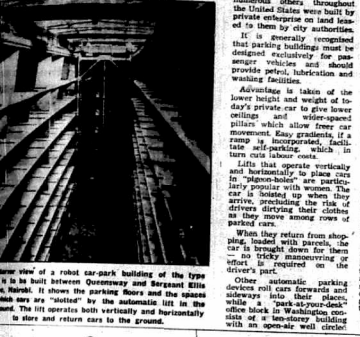
New view of a robot car-park building of the type to be built between Queenway and Sergeant Ellis Avenue, Nairobi. It shows the parking floors and the spaces which are "filled" by the automatic lift in the ground. The lift operates both vertically and horizontally to store and return cars to the ground.
