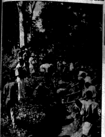
It washed away by the rains along the side of the Kirigara turrrow in the Meru district is removed by a work party to allow the water to flow through one more.
