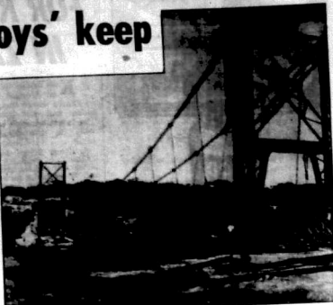
Millennium Bridge is one of several where the Materials Branch was called on to assist in foundation investigations. The supports for this particular bridge proved tricky engineering problems caused by unstable and where the anchor blocks were to be erected.
