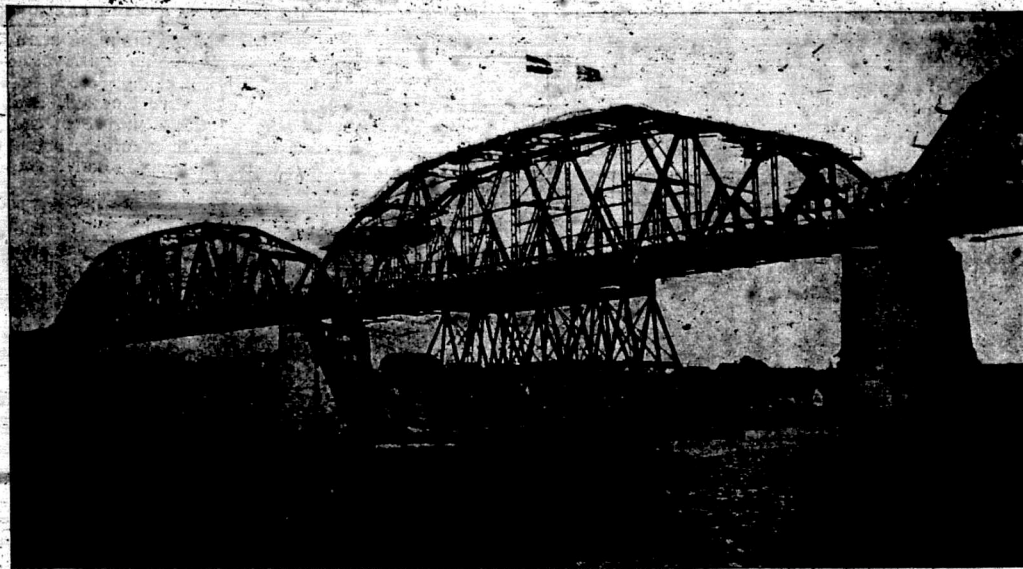
Combined Road and Railway Bridge spanning the River Daugava for the Latvian Government. It consists of three spans each of 270 feet.
