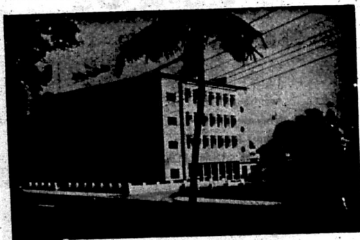
The Offices of the Company's East Africa Headquarters at Mombasa
