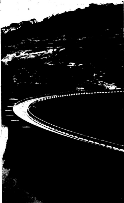
The Kyle Dam. Tribute to Rhodesian skill, both black and white, and centre of a vast irrigation scheme to cultivate the lowveld.
