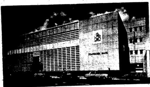
The Standard Bank in Salisbury was recently completed by Richard Costain (Africa) Ltd.
